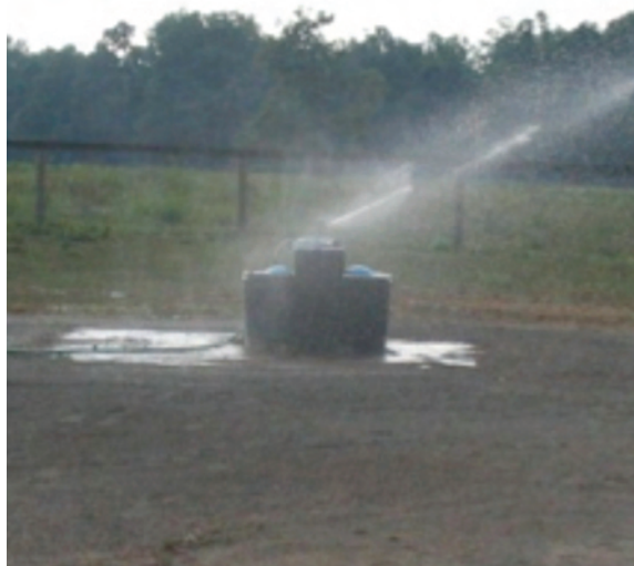
Figure 4. A 360-degree sprinkler is one way to keep the soil-cement wet.
