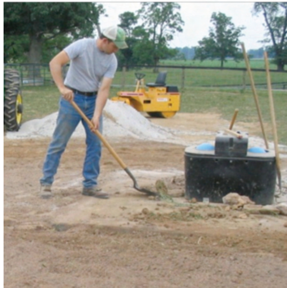
Figure 3. Rock, soil, and cement have been mixed. Notice the remaining organic matter is being removed.
