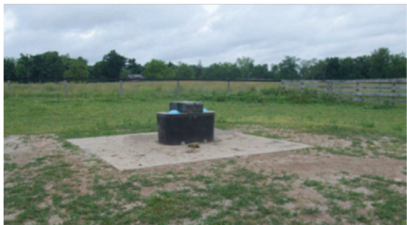
Figure 2. Shows the stability and wear of a watering pad area that was treated with soil cement two years prior.
